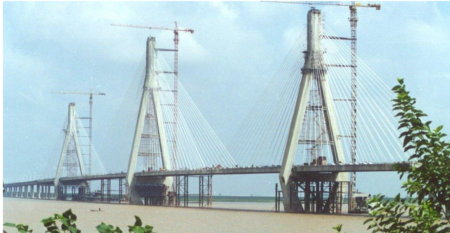
Figure 17. The Dongting Lake Bridge equipped with MR dampers in China [64]
