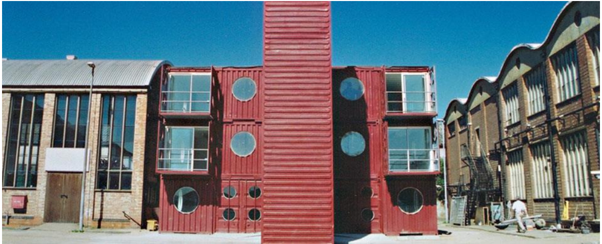
Obr. 17: Container City I
