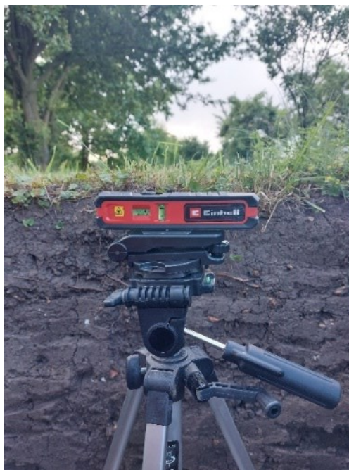
Figure 53. Using the EINHELL TC – LL 1 Classic laser spirit level during excavation.
