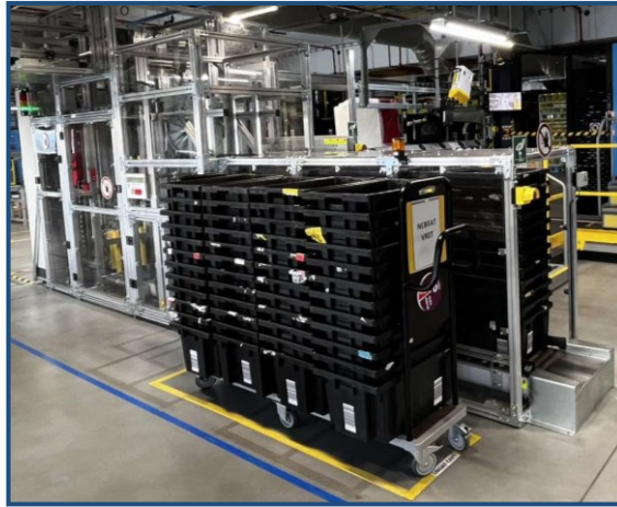
Figure 21 Totes Multi-Stacker behind full U-boat- Front view (Source: own elaboration)
